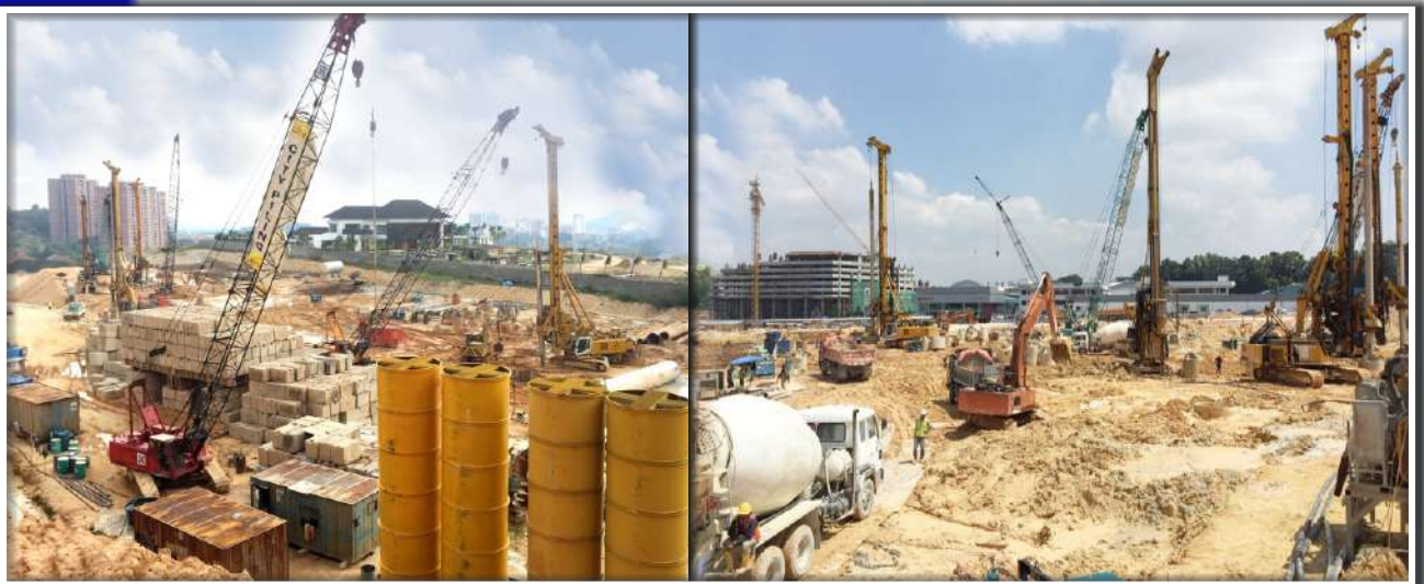
2014 CPC65 _ MRT, Saujana Impian Station
