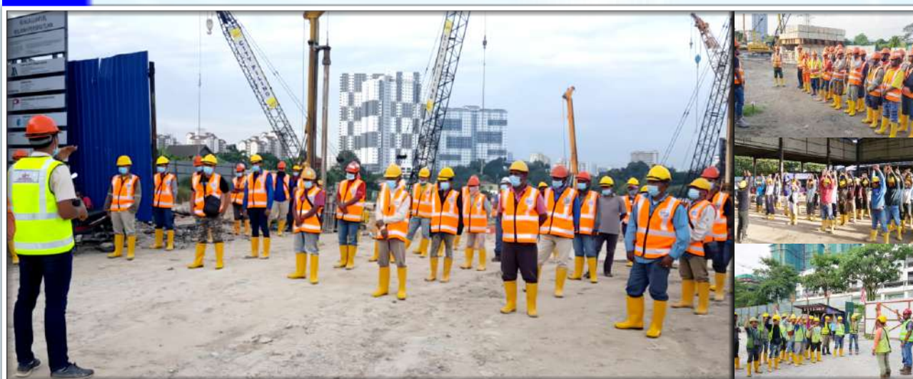
SAFETY Toolbox Meeting (TBM)_ We Practice And Adhere To Safe And Healthy Working Attitude. We Conduct TBM At Every Site With Everyone Involved.
