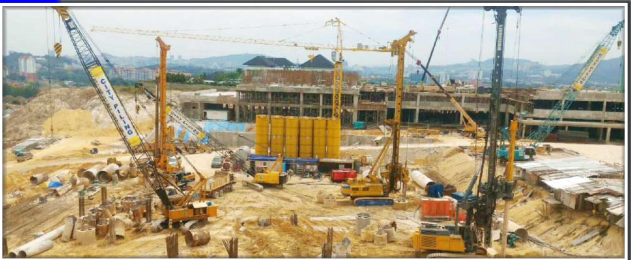
2016 CPC80 _ Bridge For City Of Green @ Bukit Serdang Apartment
