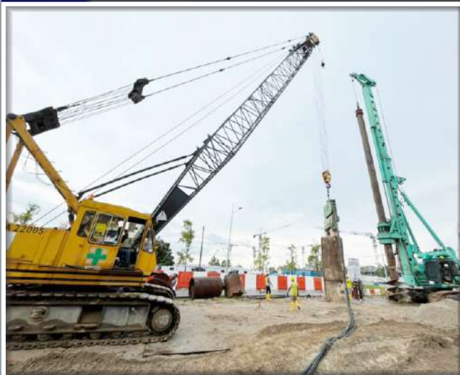
2022 CPC129 _ Lim Chong Eu Bridge, Penang
