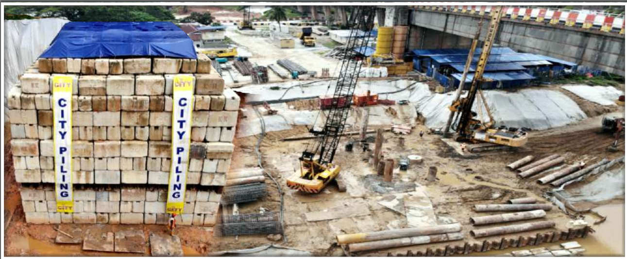
2021 CPC171 _ Shas Bridge, Temerloh, Pahang
