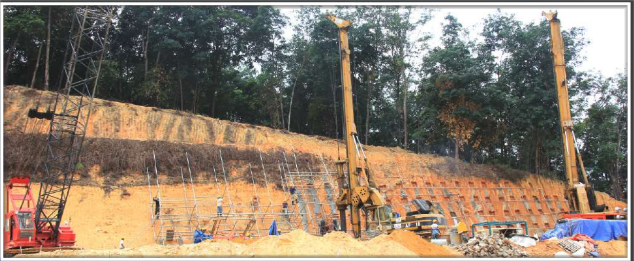
2014 CPC67 _ Damai Hillpark @ Desa Cheras (Slope Stabilisation Works)
