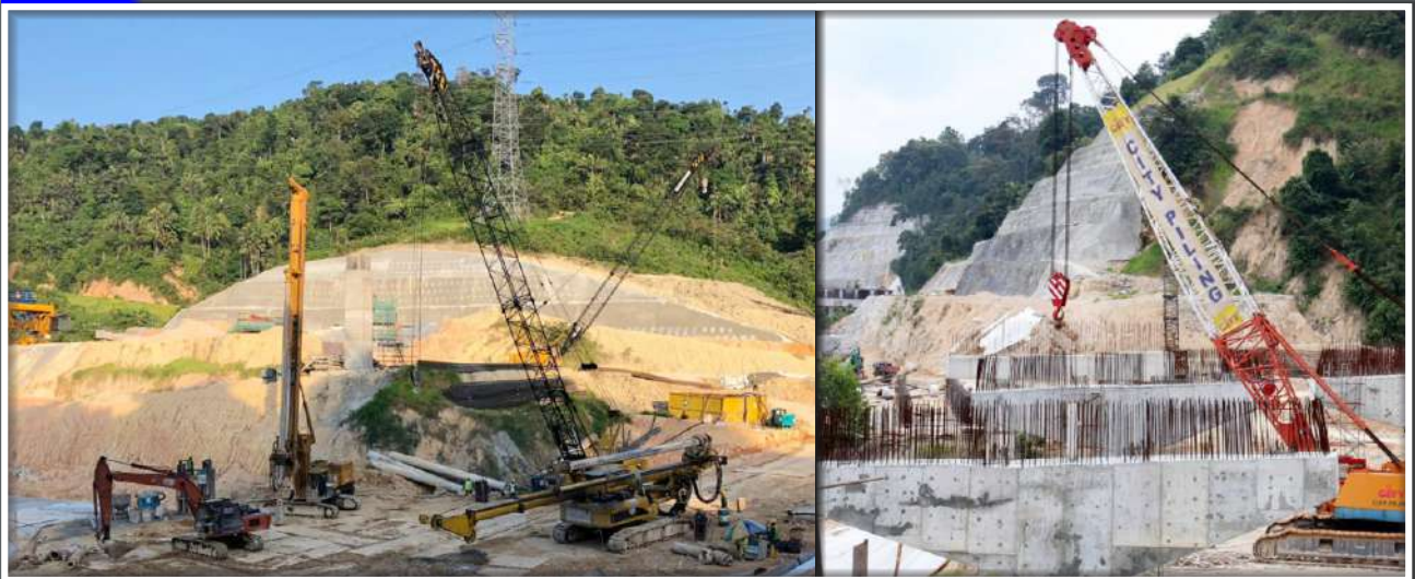
2018/19 CPC102, 105, 106 & 109_ Suke Highway, Package CB1, Viaduct 1, 1A, 2A, 3, 4 & CBP Wall
