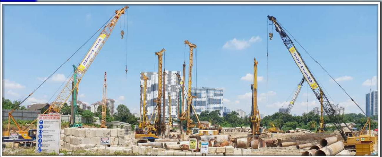
2020 CPC115_ (PPAM) @ Setapak Riviera (Bored Pile)
