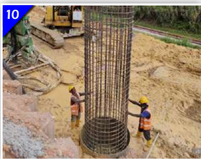
10 Prefabricated Reinforcement Steel Cage Is Then Installed Into The Bored Hole.
