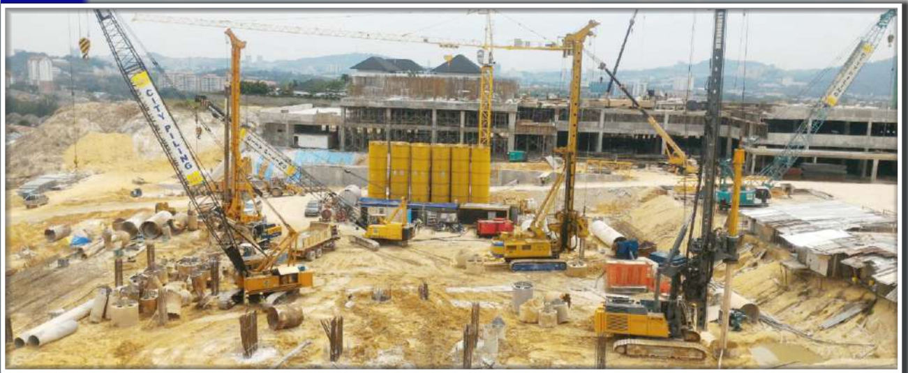
2013 CPC59 _ City Of Green @ Bukit Serdang (Bored Pile)
