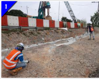
1 Firstly, Qualified Land Surveyor Set Out The Intended Bored Pile Point.
